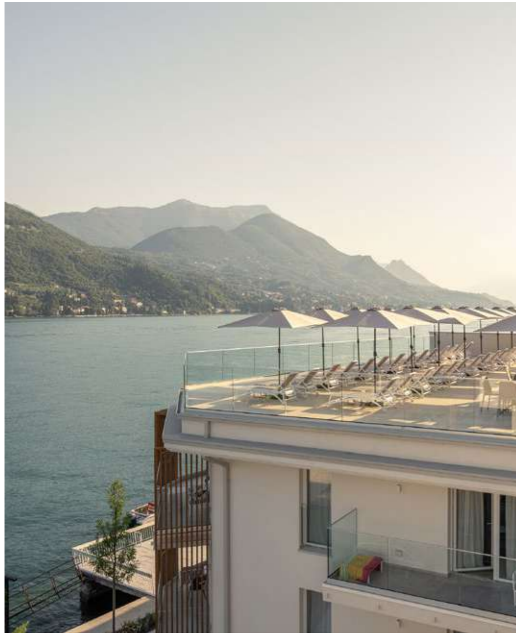
AH Porticcioli Boutique Apartments Resort San Felice del Benaco - Italy Project: Hotel Products: Atlantico, Pop
